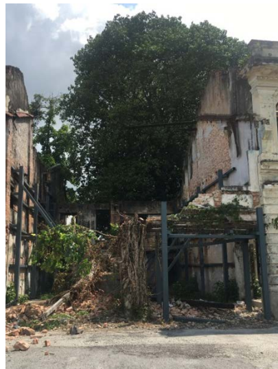
Figure 7 Shophouses A17-18 (April 2017)
