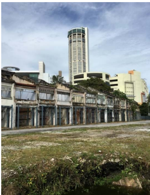
Figure 4 The second cluster of shop houses. This image shows the slight curved configuration. (January 2017)
