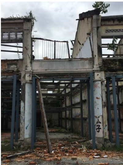
Figure 6 Shophouse A8 (January 2017)
