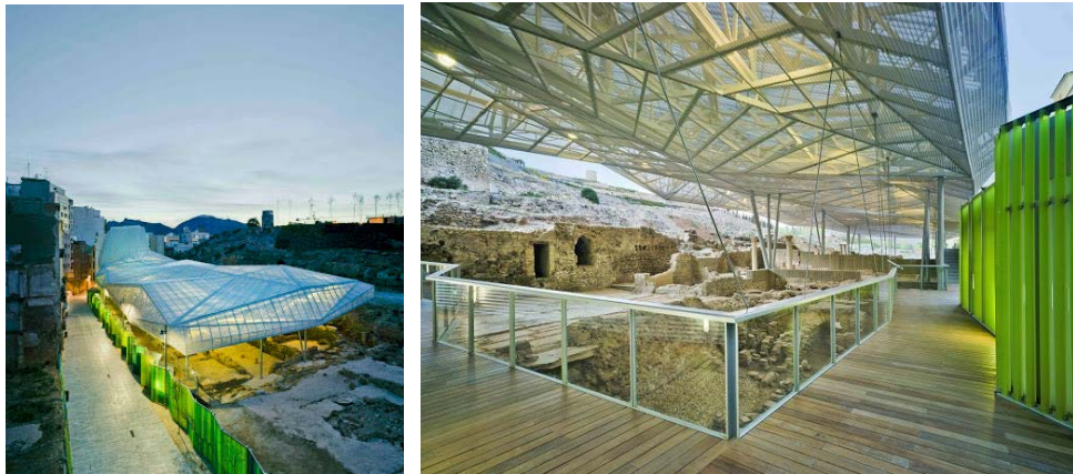
Figure 21 These roman ruins in Cartagena, Spain, are several meters below the current road level. A deck was built around them and a modern protective cover installed over them in 2011.
