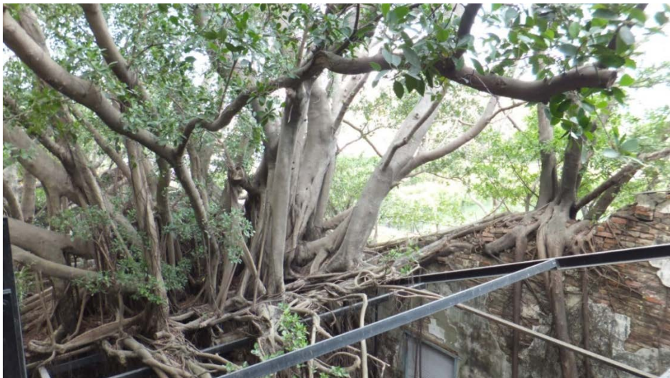
Figure 25 The roof of the "Tree House" in Taiwan
