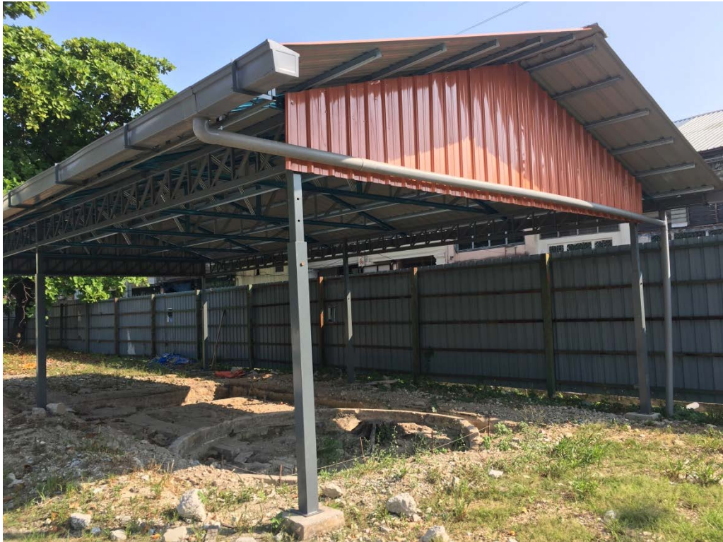
Figure 13 The new semi-permanent structure over Site B.
