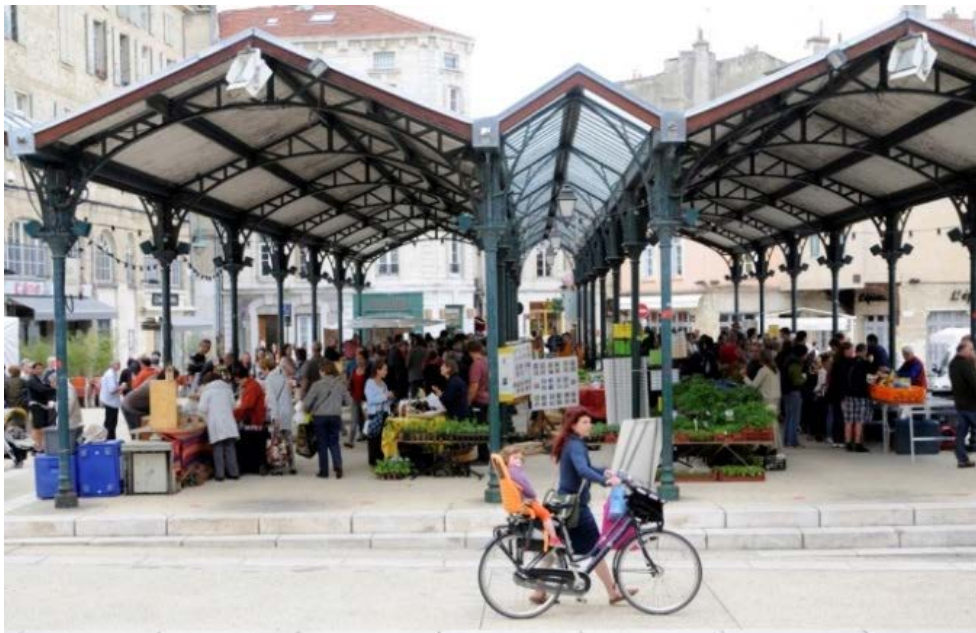
Figure 17 19th century cast iron market in Valence, France
