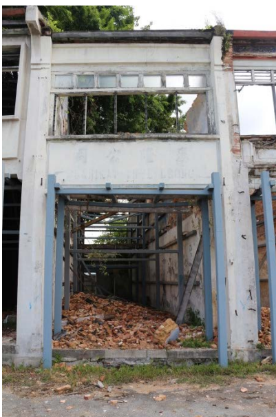
Figure 8 Shophouse A5 (October 2017)
