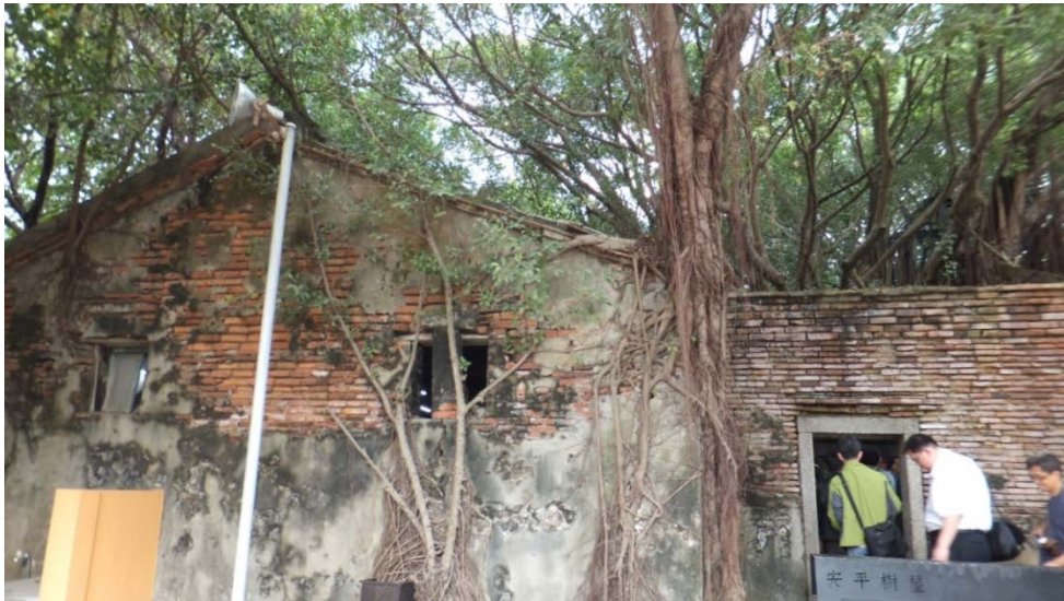
Figure 24 Side view of the "Tree House" in Taiwan
